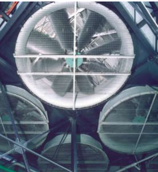
Example of an axial fan installation.
